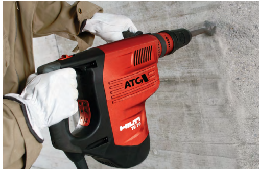
b) Surface roughening using brushing tool
