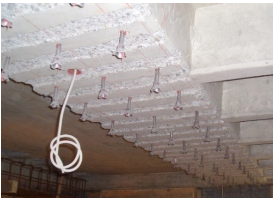
a) Increasing RC beam depth
