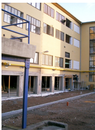
a) The 3 storey industrial building
