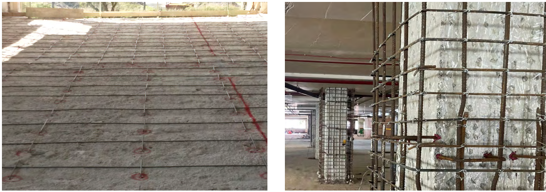
g) Slab shear-friction overlay
