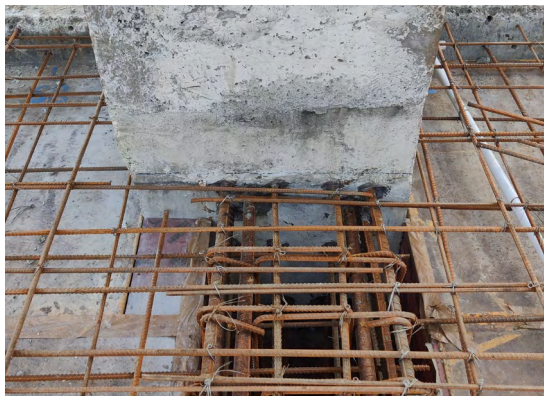
d) Beam-to-column connection
