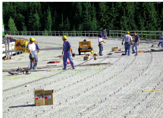
d) Increasing bridge deck slab thickness
