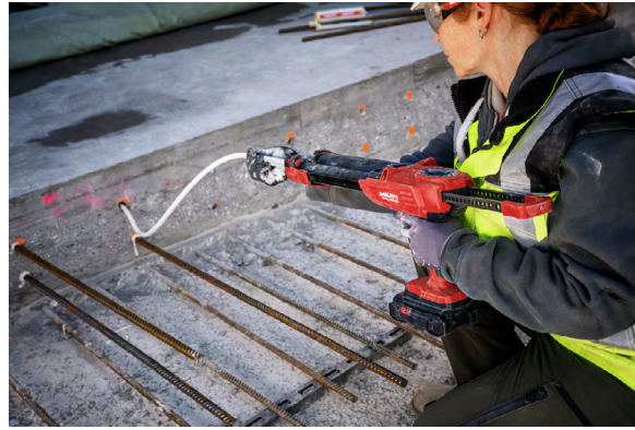
b) Extension hose for adhesive mortar injection
