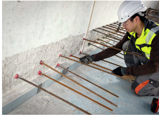
b) Slab-to-wall connection
