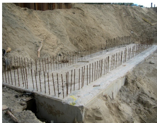
c) Abutment structure with post-installed rebars
