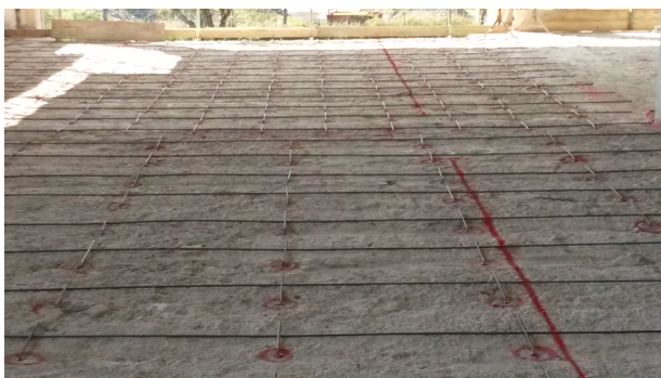
a) Concrete overlay on existing floors
