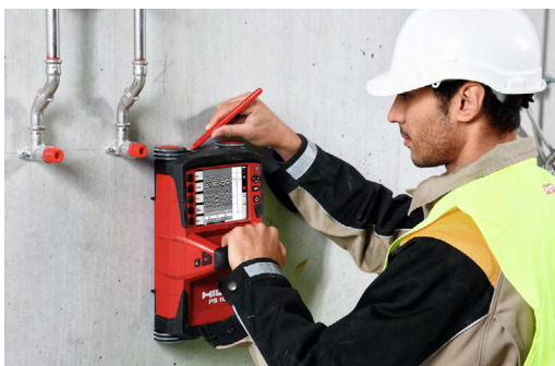
c) Scanning for ferrous & non-ferrous objects
