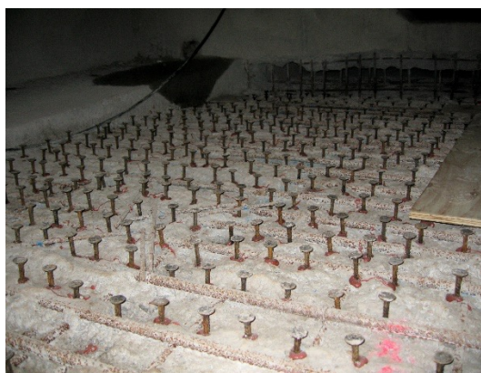
b) Bridge box-girder strengthening with HCC-K shear connectors
