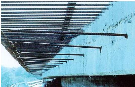
Post-installed rebar connections in infrastructure requalifications Slab widening
