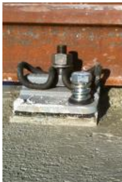
Support after concrete pouring
