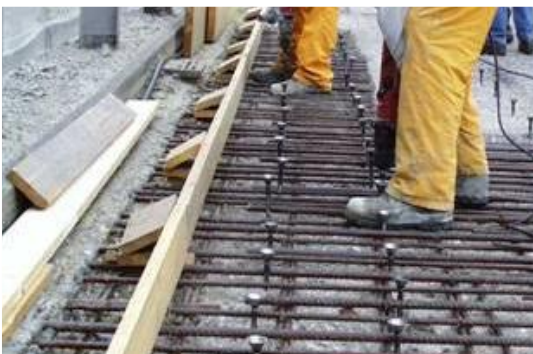
Slab strengthening
