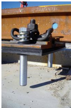
Clipped components before concrete pouring
