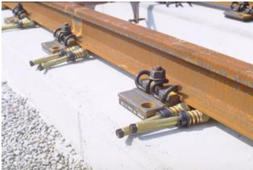
Bottom-up construction method
