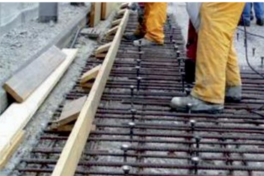
Slab strengthening
